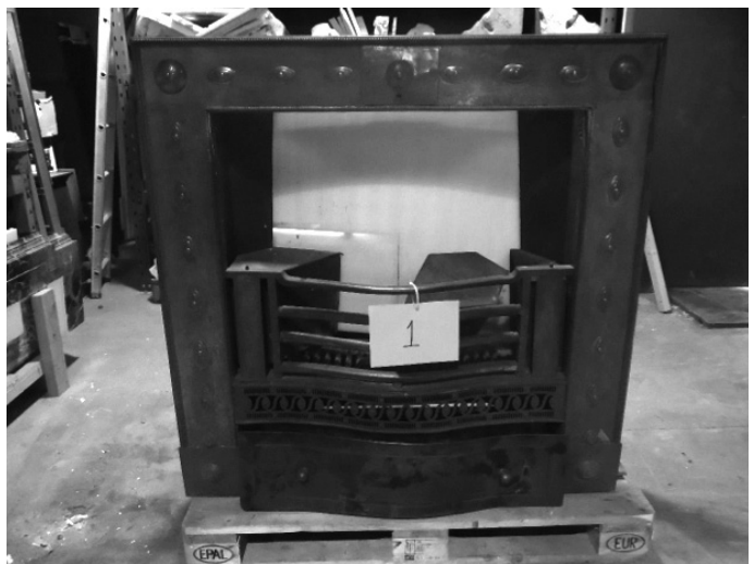
Original register grate in steel, provenance as above.
